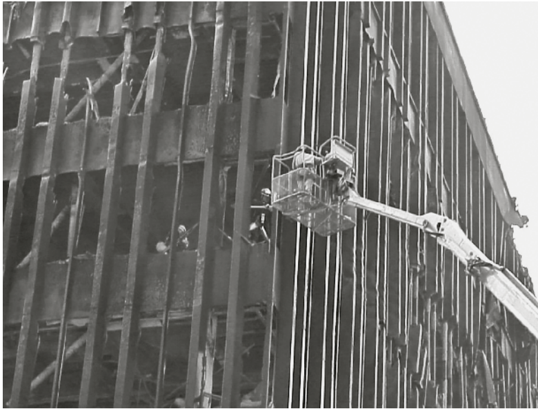
Miles, along with a FEMA Search Dog Handler (and a search dog), on the way up to search Building 4. Entry from the ground was impossible due to the stairwell being destroyed.
